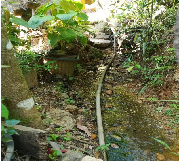
Figure 04 (a) – Water runs through a house due to non-availability of drainage system.
