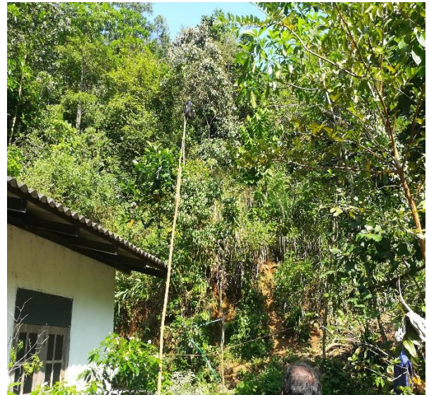
Figure 04 (b) – Vegetation surrounding the slope
